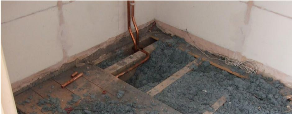
Loose fill blue asbestos insulation material (photo: UK Health and Safety Executive)
